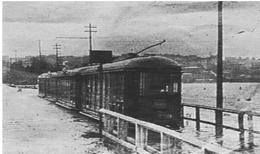
track. When minor flooding occurred, drivers were instructed not to cross the bridge or approaches when water reached a depth of 6 inches over the tracks.
